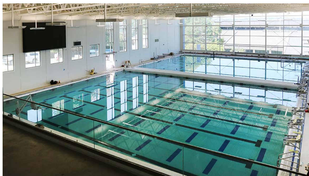
The finishing touches are being done on the new pool, slated to open this week.
